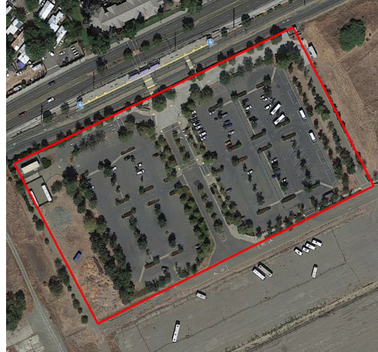
Figure 4-5 Hazel Garage - Existing Conditions
