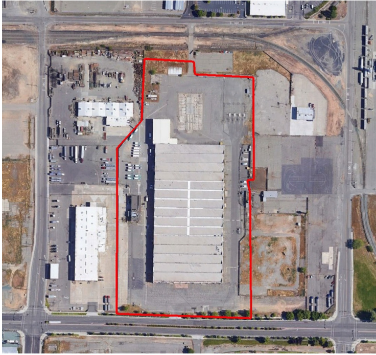
Figure 4-4 McClellan Garage - Existing Conditions | Source: WSP
